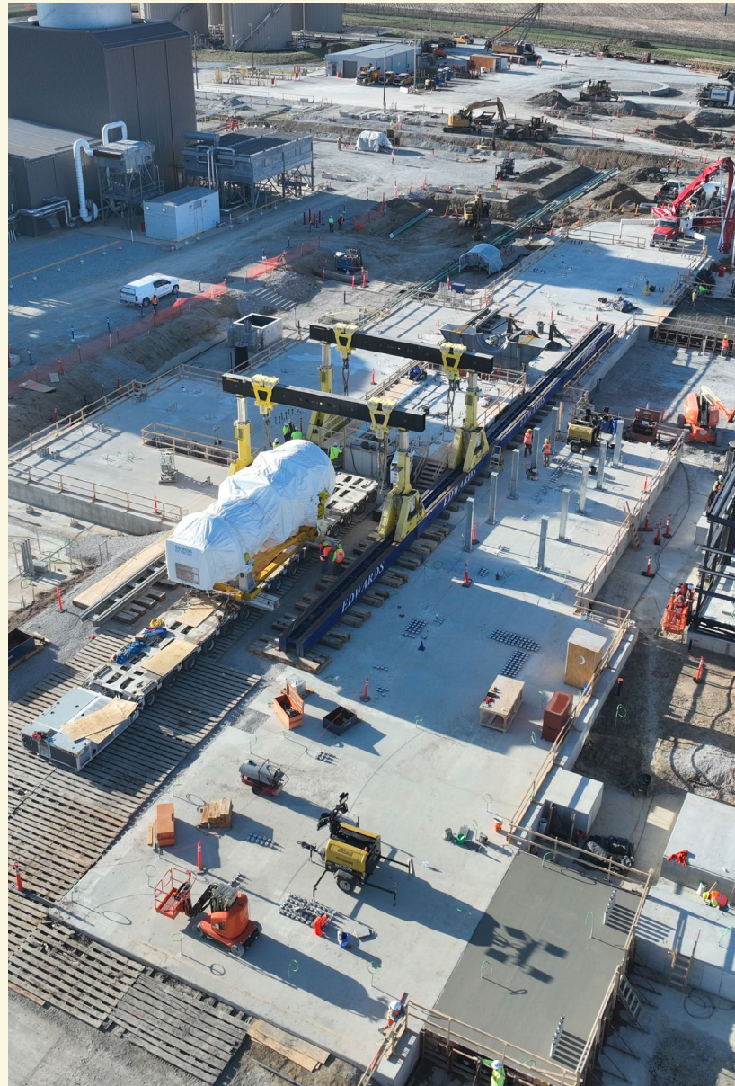
Combustion Turbine and gantry crane set up for final move into place. ➤
