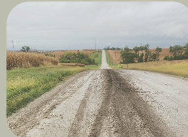
Turtle Creek Station construction activity – road construction, small footprint
