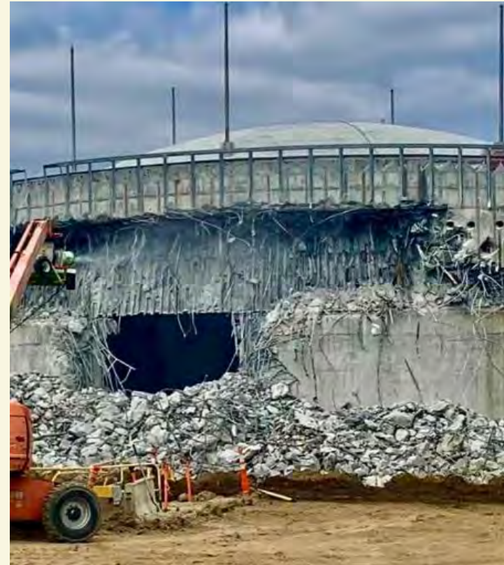
Demo Continues – Week 3
