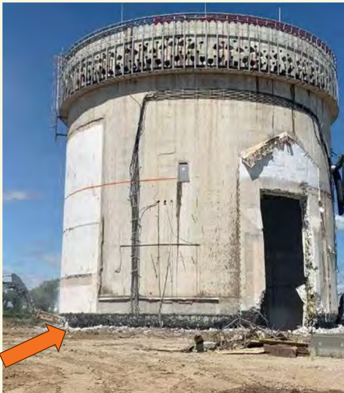
Containment Demolition Begins (8/25/25)
