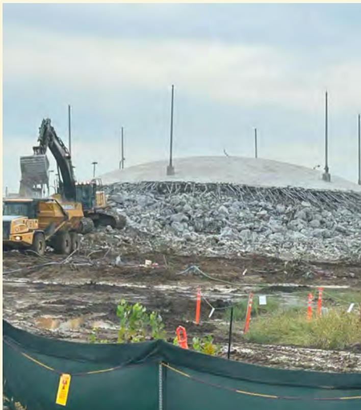
Demo Continues – Week 4
