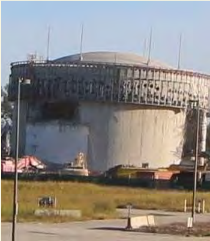
Demo Continues – Week 2
