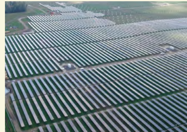
Pierce County Energy Center
