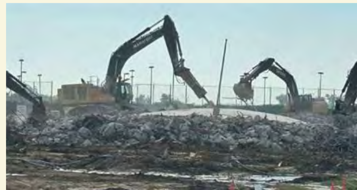
Demo Continues – Week 5
