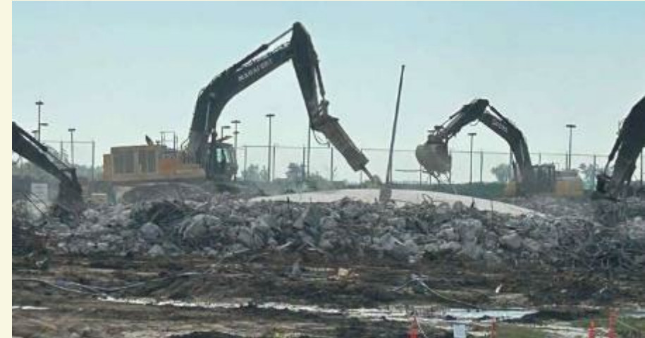
Demo Continues – Week 5
