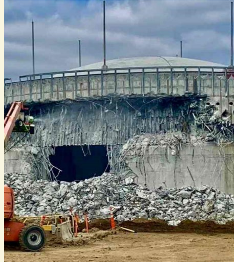
Demo Continues – Week 3
