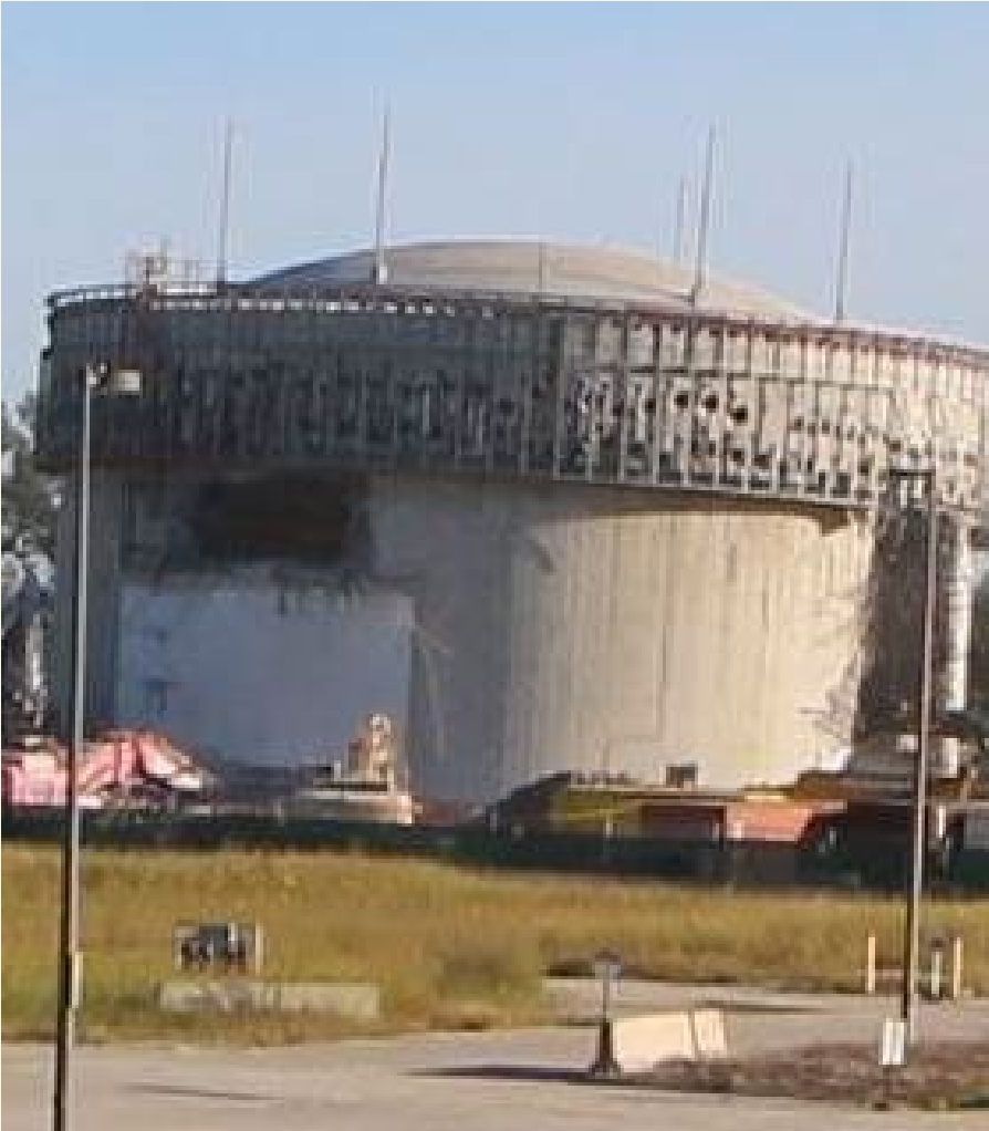
Demo Continues – Week 2
