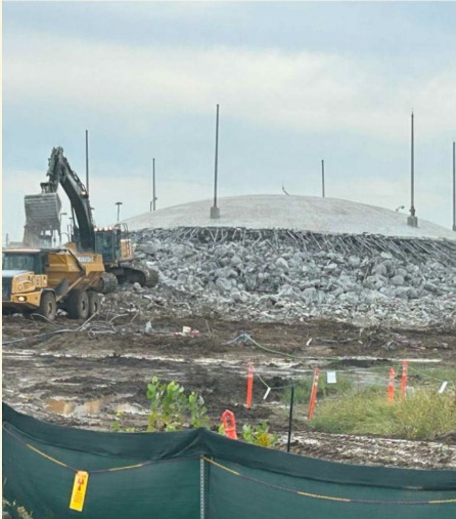
Demo Continues – Week 4
