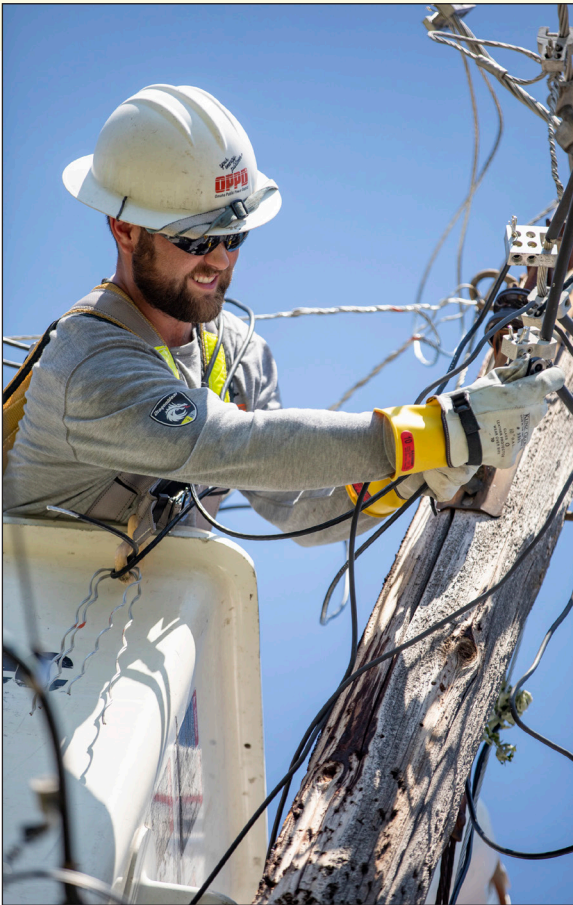
Above and top: Crews work to restore power after the July 31 windstorm that caused more than 221,000 customers to lose power.
