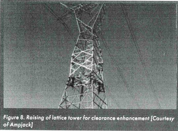
Figure 8. Raising of lattice tower for clearance enhancement [Courtesy of Ampjack]
