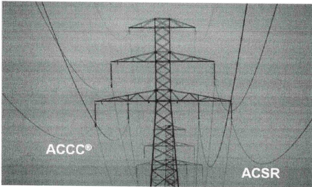
CTC Global, for example, developed an ACCC cable that has 28% more aluminum compared to an ACSR cable of the same size, which allows the cable to carry more current while suffering lower power losses [4]. The image below shows a CTC ACCC cable compared to a traditional ACSR cable of same size.
