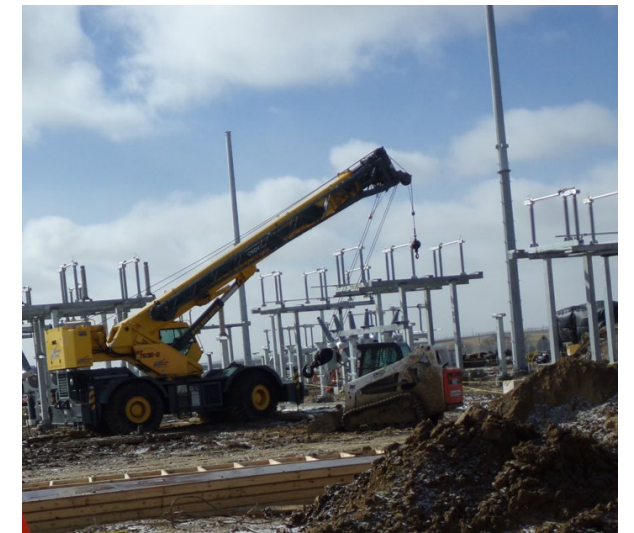
Substation Switch Installation
