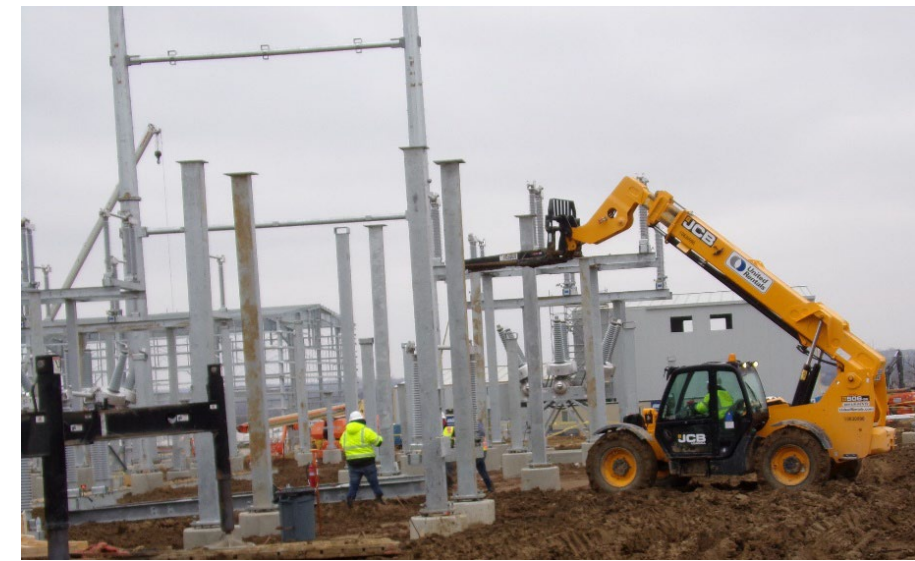
Facing West – Substation H-Frame & Switch Placement
