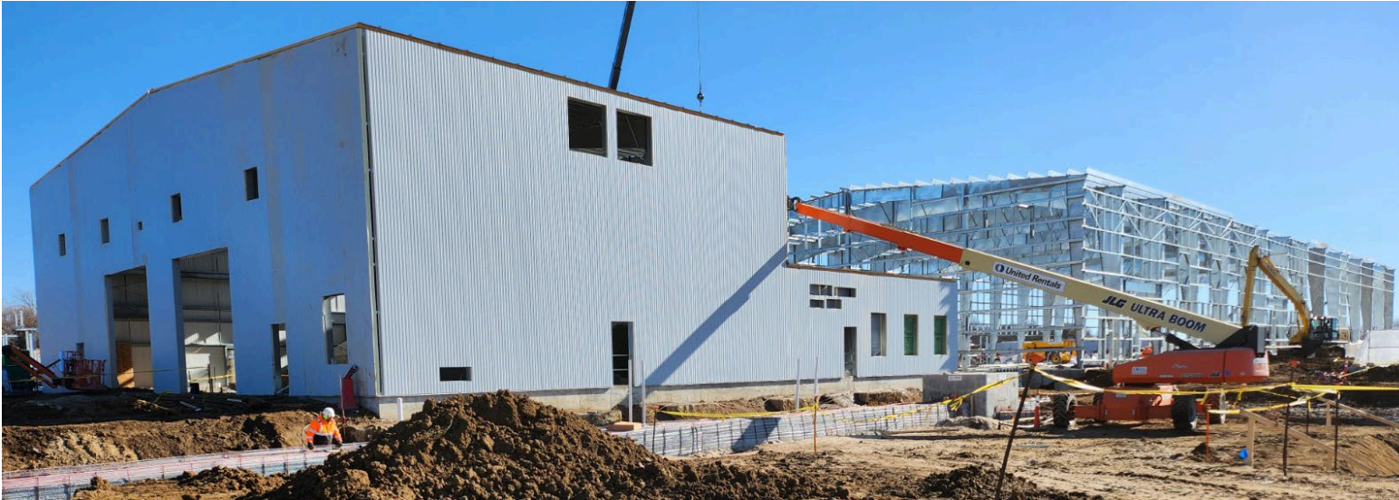
Facing Southeast – Engine Hall & Administrative Building Enclosures
