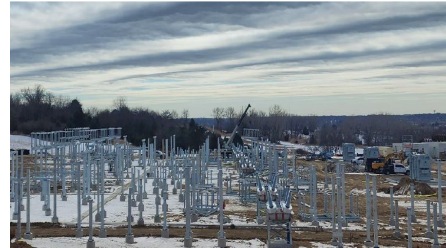
Facing South – Switchyard Erection
