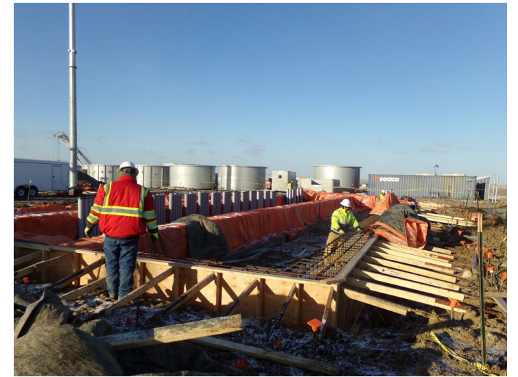
Substation Control House Foundation Preparation
