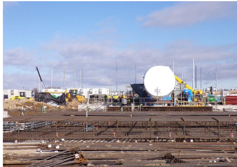
Facing North – Unit #2 Stack Foundation Prep
