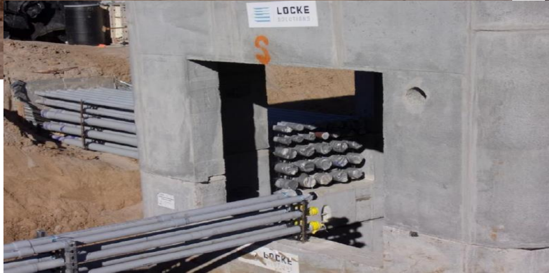
Manhole Penetrations
