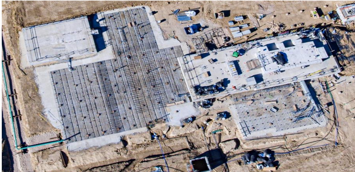
Unit #1 Generator/Gas Turbine at TCS site
