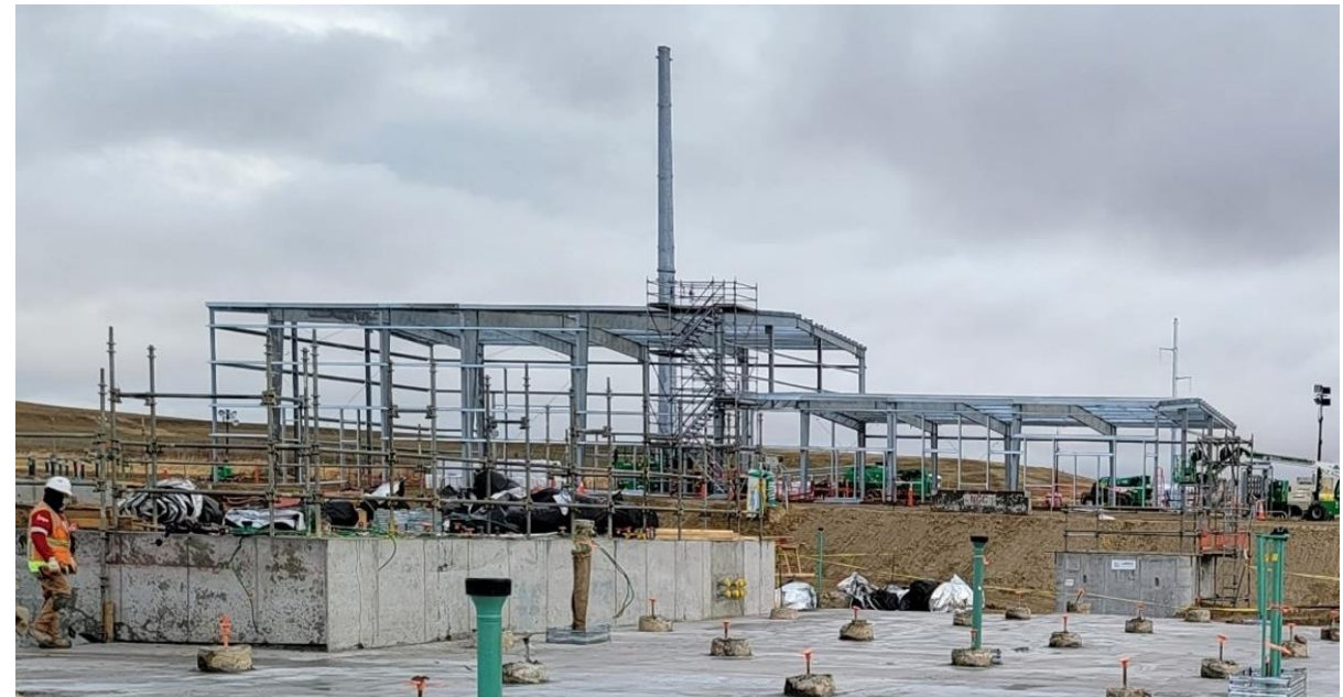
Facing East – Unit 1 with Admin Building
