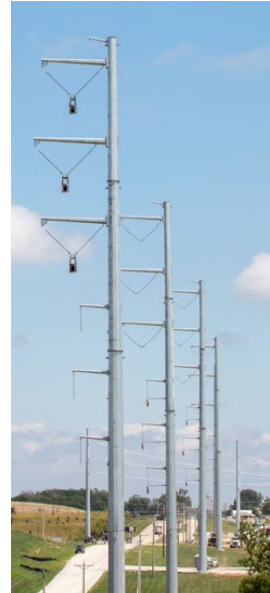
Double Circuit 345/161kV
