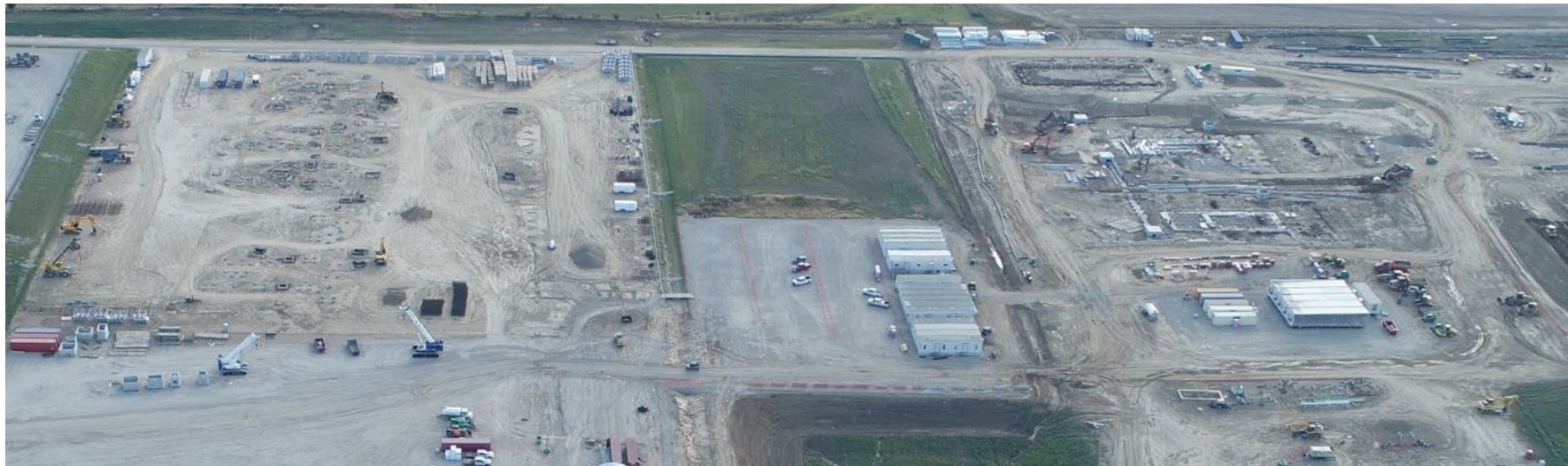
Facing East – Aerial view of substation and production sites on 10/2/2022
