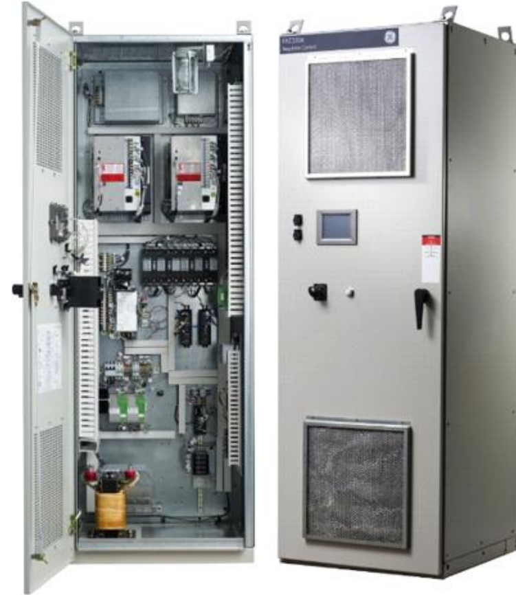
EX2100e Control Cabinet (35 A Regulator System)
