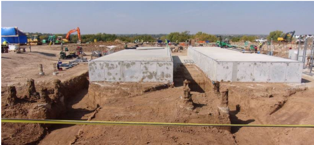
Facing West - Engine Foundations 1 & 2 on 10/9/2022
