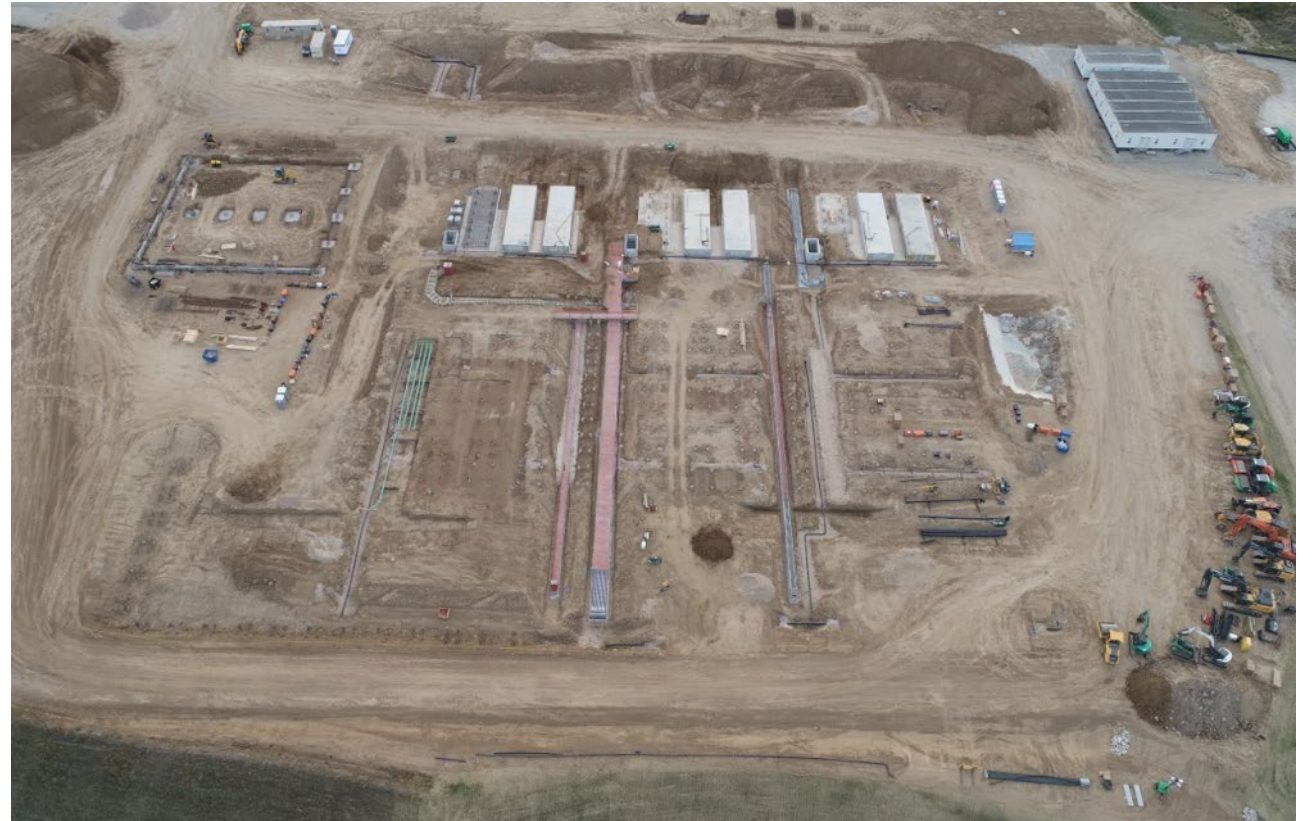
Facing East - Aerial view of generation area on 9/18/2022
