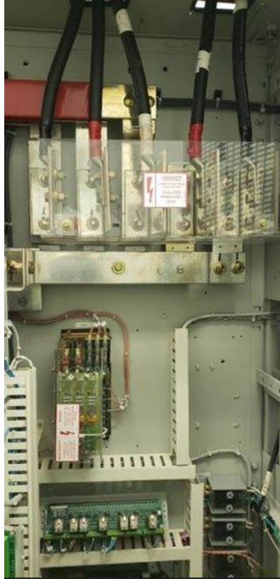
Representative Existing Exciter Hardware
