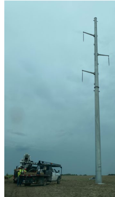
Single Circuit 161kV
