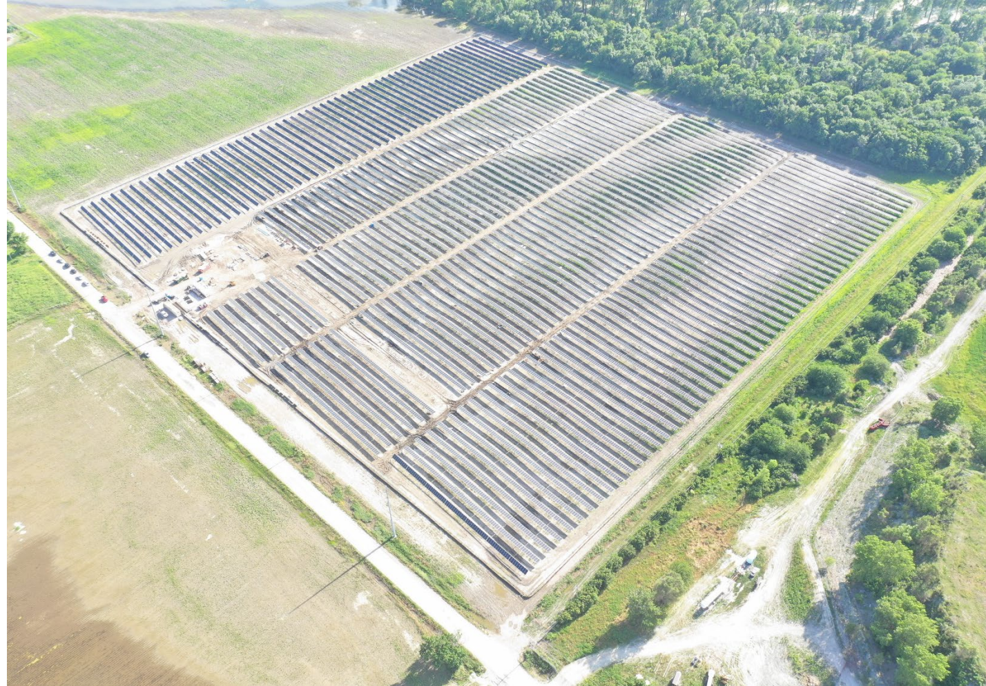
Photo: Fort Calhoun Community Solar drone footage
