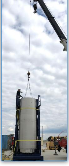
Each canister weighs 46,000 pounds empty. Material and weld inspections ensured canisters were undamaged during transport.
