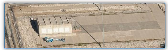
Crews expanded the Independent Spent Fuel Storage Installation (ISFSI) from 10 original Horizontal Storage Modules (HSMs) to 42
