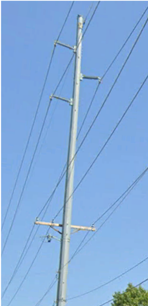
Steel Transmission Pole
