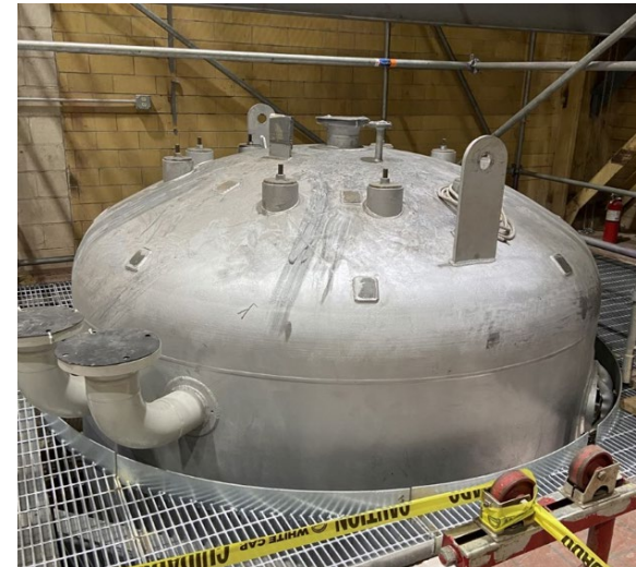
Auxiliary Boiler set in place
