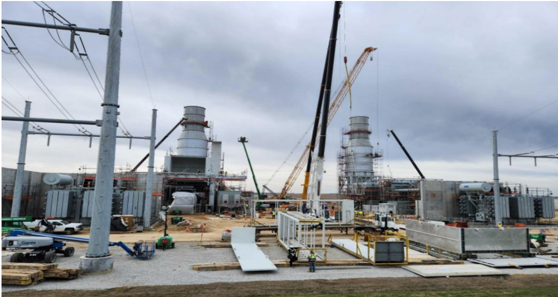
Facing South – Power Block Progress
