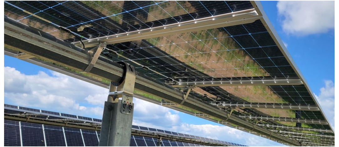
Platteview Solar – Racking & Module Installation
