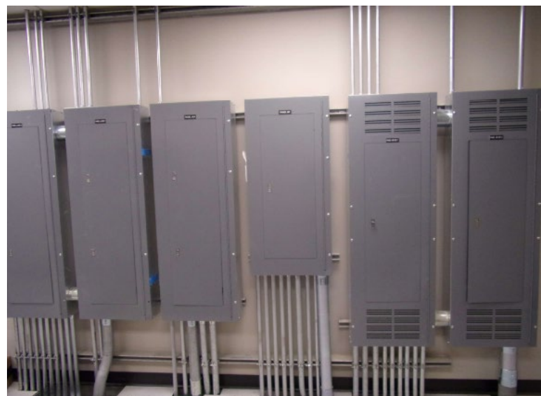
Distributed Control System Panels/Room
