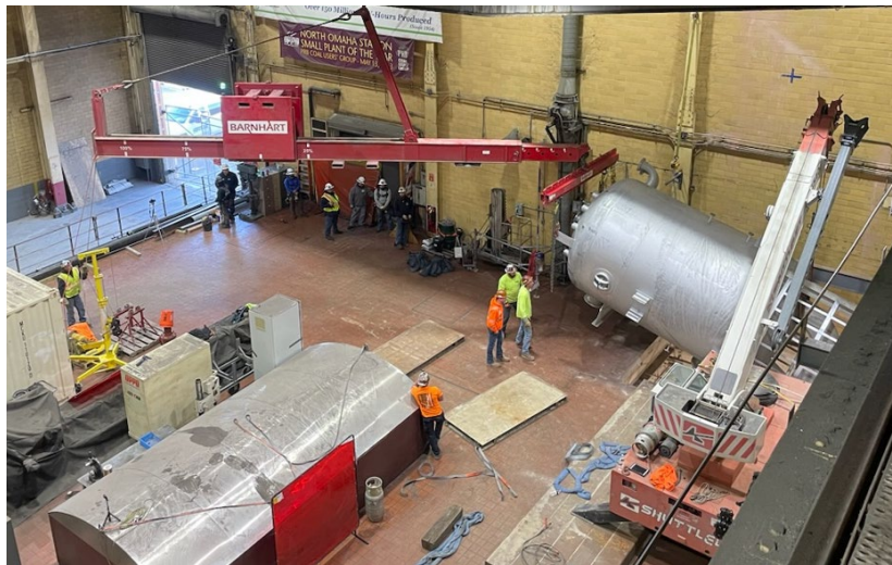
Auxiliary Boiler upending
