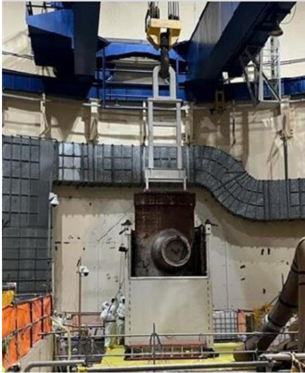
Placing in Shipping Container
