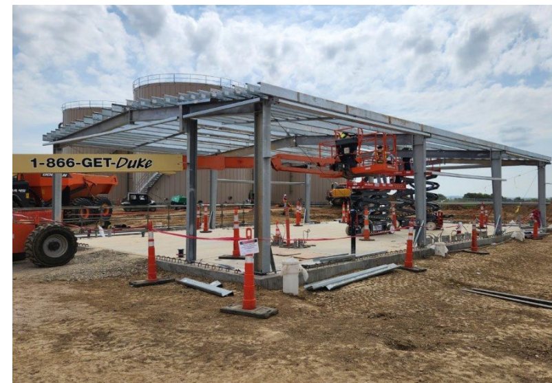
Fuel Building Erection
