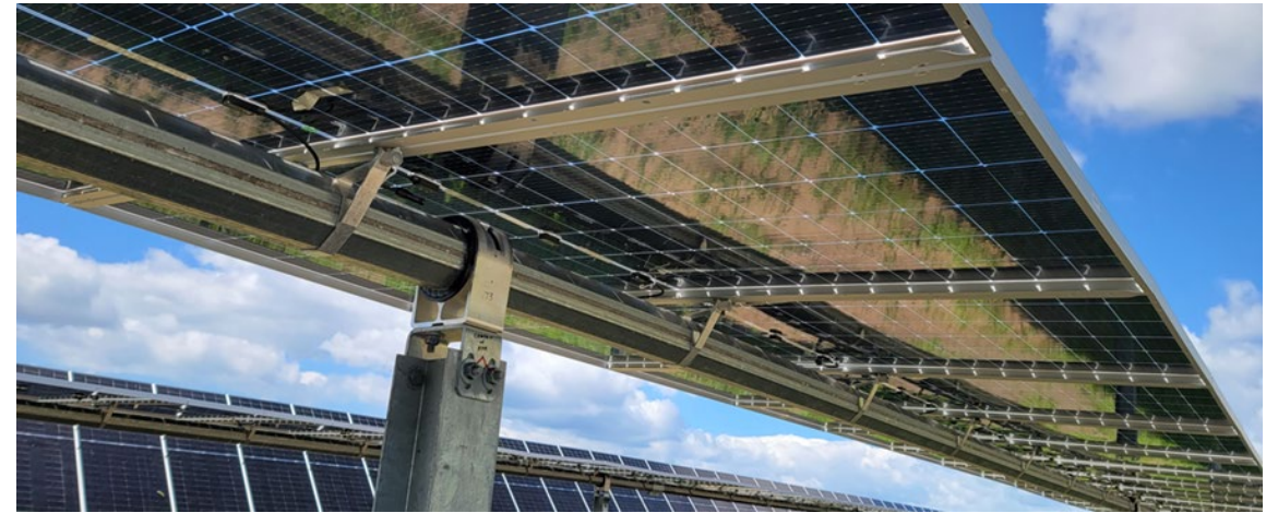
Platteview Solar – Racking & Module Installation
