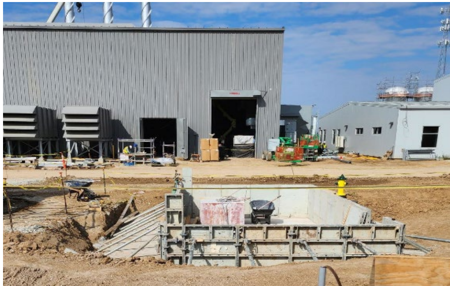
Facing West – Emergency Diesel Generator Foundation
