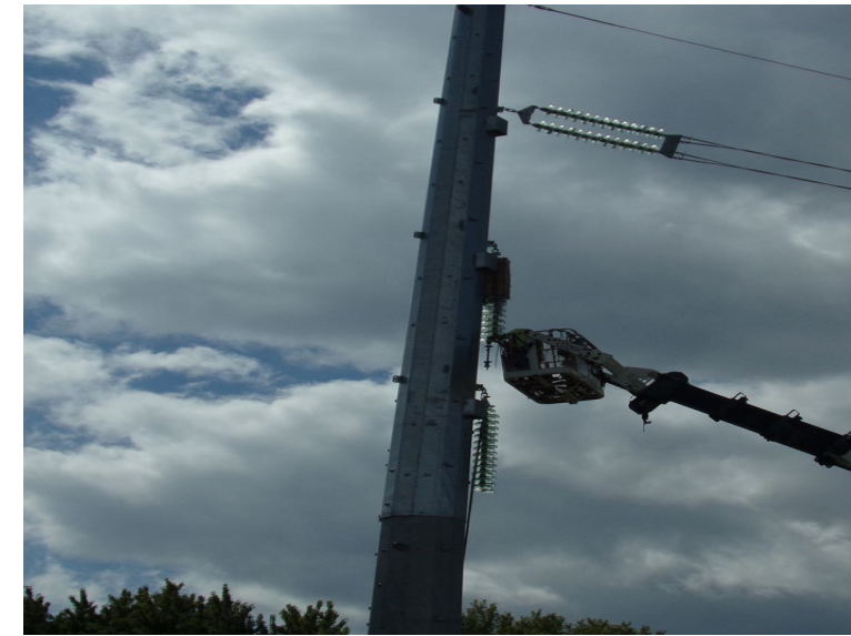
Substation Static Cable Mast Install
