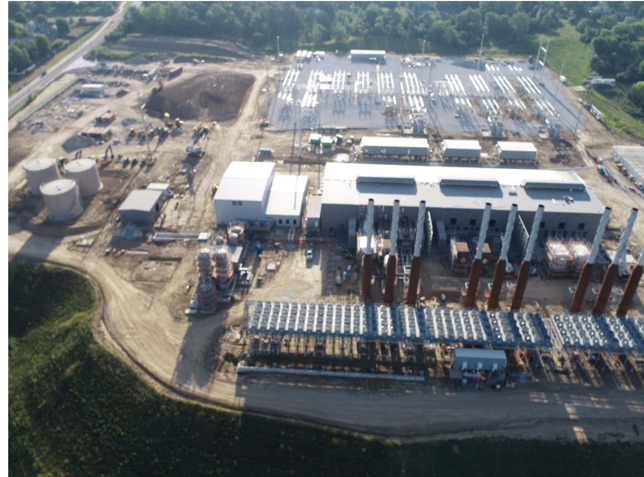
Facing East – Aerial SBLs, September 2023
