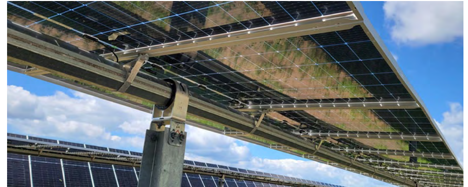
Platteview Solar – Racking & Module Installation
