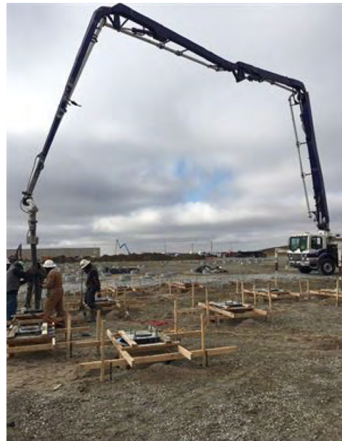
Pier Formwork
