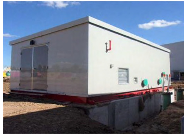
Facing Southeast - Fire Water Pump House
