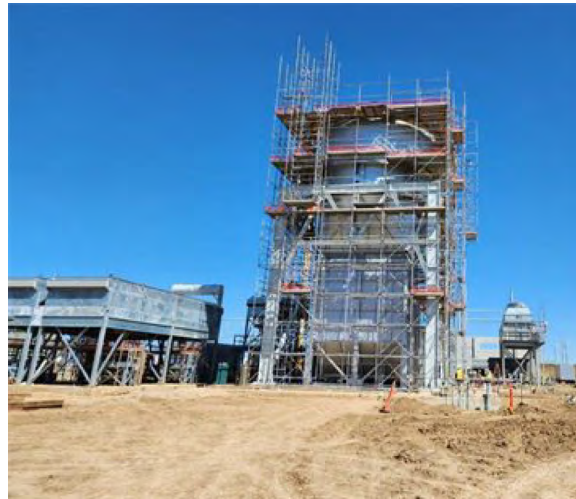
Facing North- Unit #1 Stack Erection
