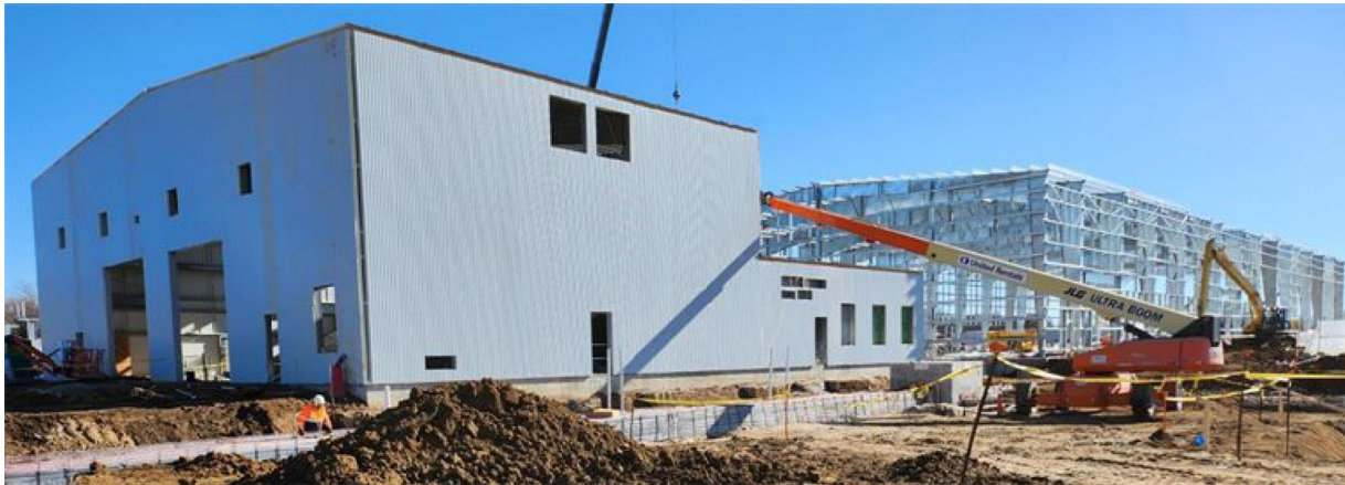
Facing Southeast – Engine Hall & Administrative Building Enclosures
