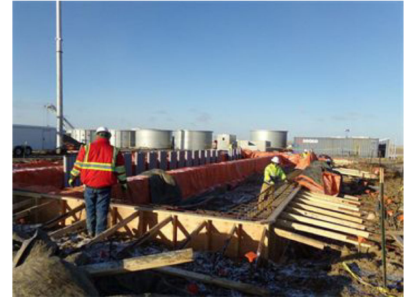
Substation Control House Foundation Preparation
