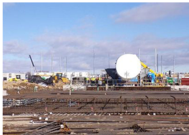
Facing North – Unit #2 Stack Foundation Prep
