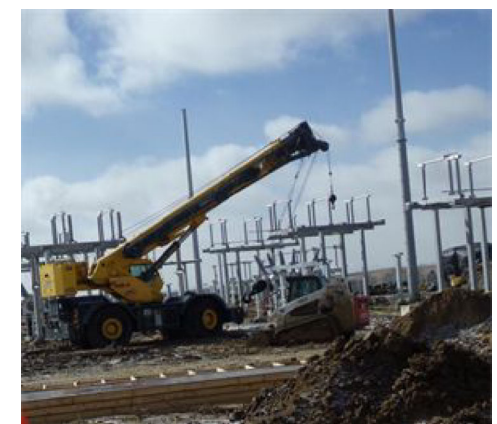
Substation Switch Installation
