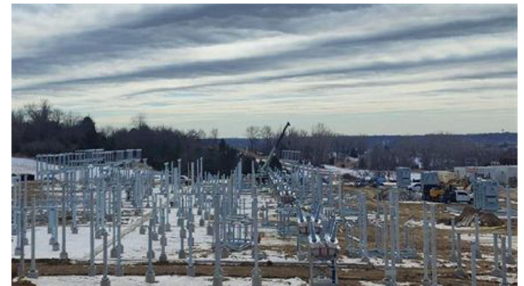
Facing South – Switchyard Erection
