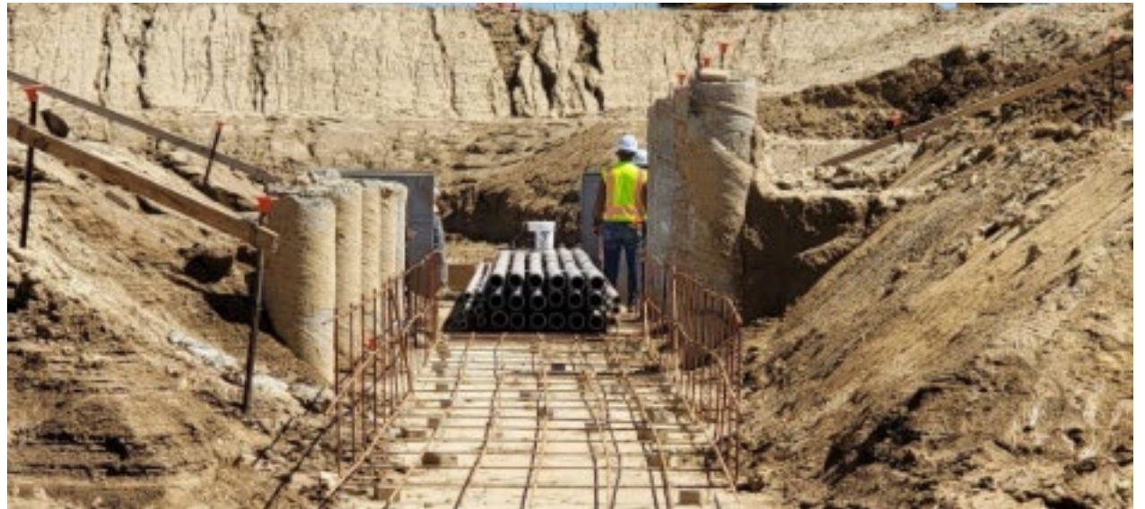
Facing East – Install Conduit Duct Bank
