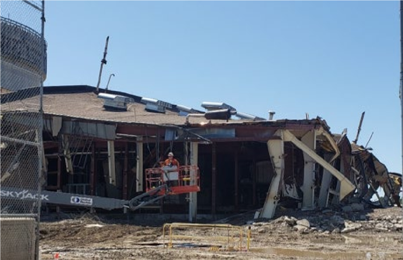
Turbine Building Upper Portion Demo Begun
