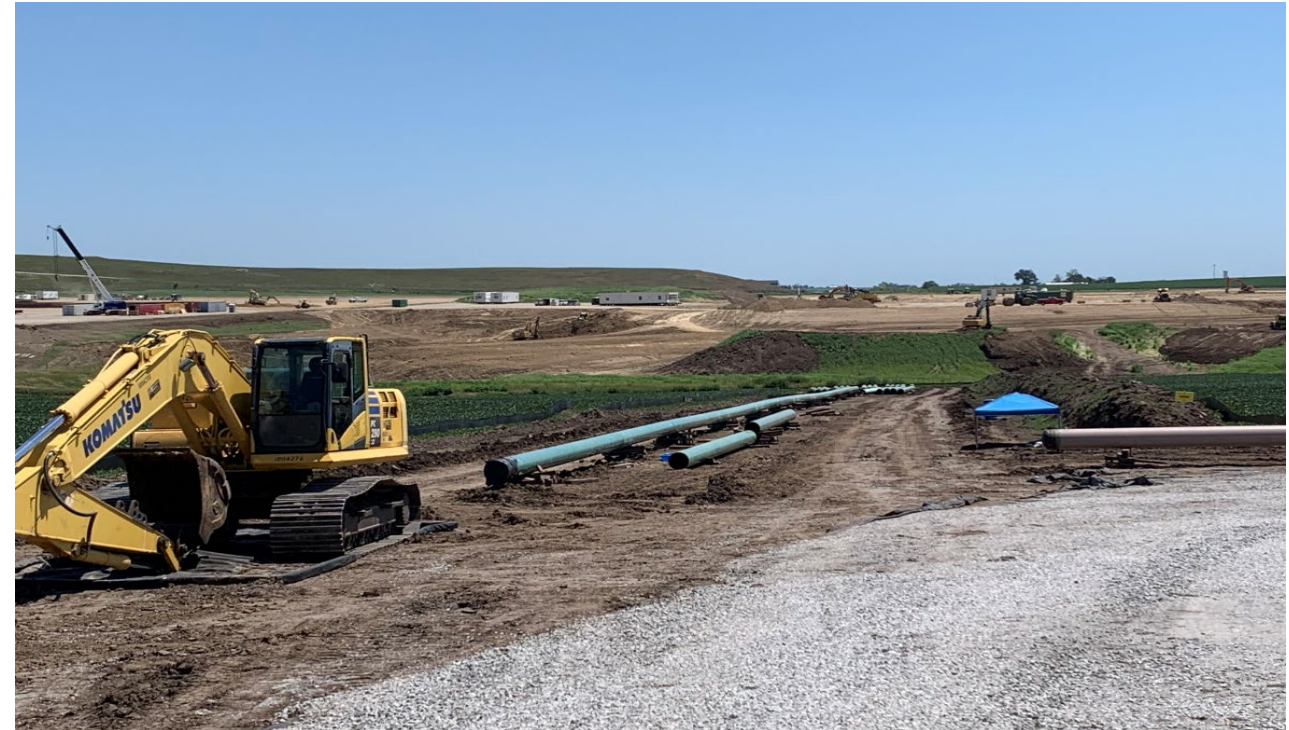
(Site pipeline construction, Looking East)
