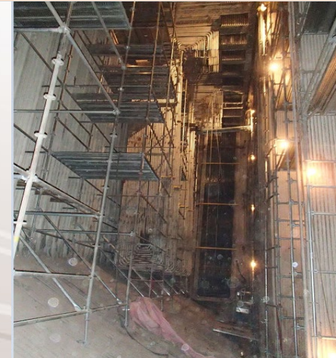
NC1 furnace slope replacement project
