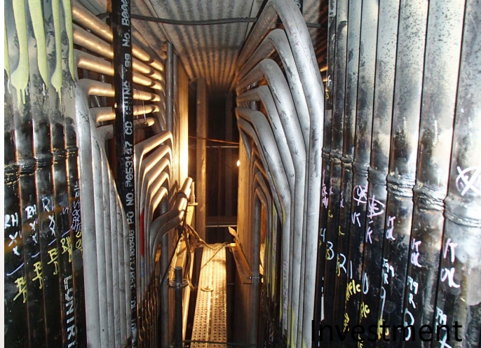
NC1 finishing superheat replacement
