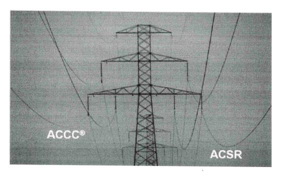
CTC Global, for example, developed an ACCC cable that has 28% more aluminum compared to an ACSR cable of the same size, which allows the cable to carry more current while suffering lower power losses [4]. The image below shows a CTC ACCC cable compared to a traditional ACSR cable of same size.
