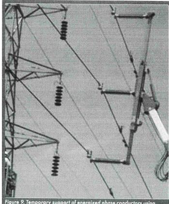
Figure 9. Temporary support of energized phase conductors using insulated crane mounted lift [6]
